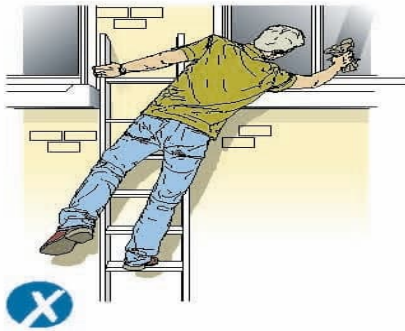
Figure 1a Incorrect - overreaching and not maintaining three points of contact
